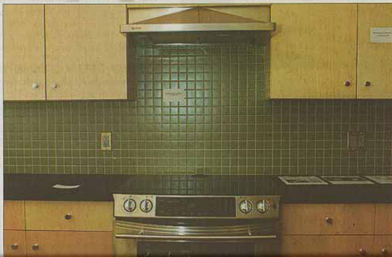
The 1,900-square-foot house features a kitchen that includes Energy Star-rated appliances, formaldehyde-free cabinets and countertop made of recycled glass and cement.
