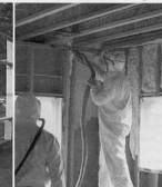
Workers apply a soy-based foam insulation into the home's walls.
