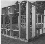
The house's frame uses carefully-placed planks to reduce overall wood use.
