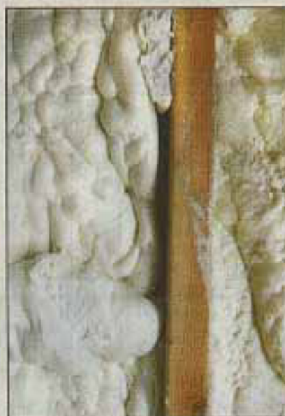
(Top) An 1,850-square-foot home under construction on Valley Road will use 50 to 80 percent less energy than a typical home. (Above) Architect Russ Hamlet, developer Lisa Martin and builder Geoffrey Hobert look over the soy-based foam insulation (above right) that is one of the key components to the efficiency of the house.
